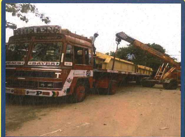
TRANSPORTATION WITH MOBILE CRANE OUTSIDE WORK
