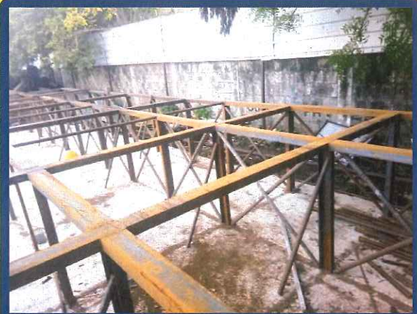
ON SITE STRUCTURAL FABRICATION
