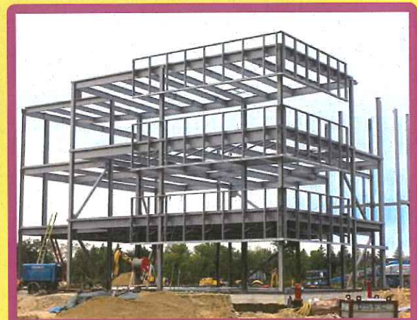
ON SITE FABRICATION STRUCTURAL
