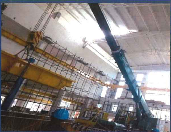
EOT CRANE ERECTION & COMMISSIONING
